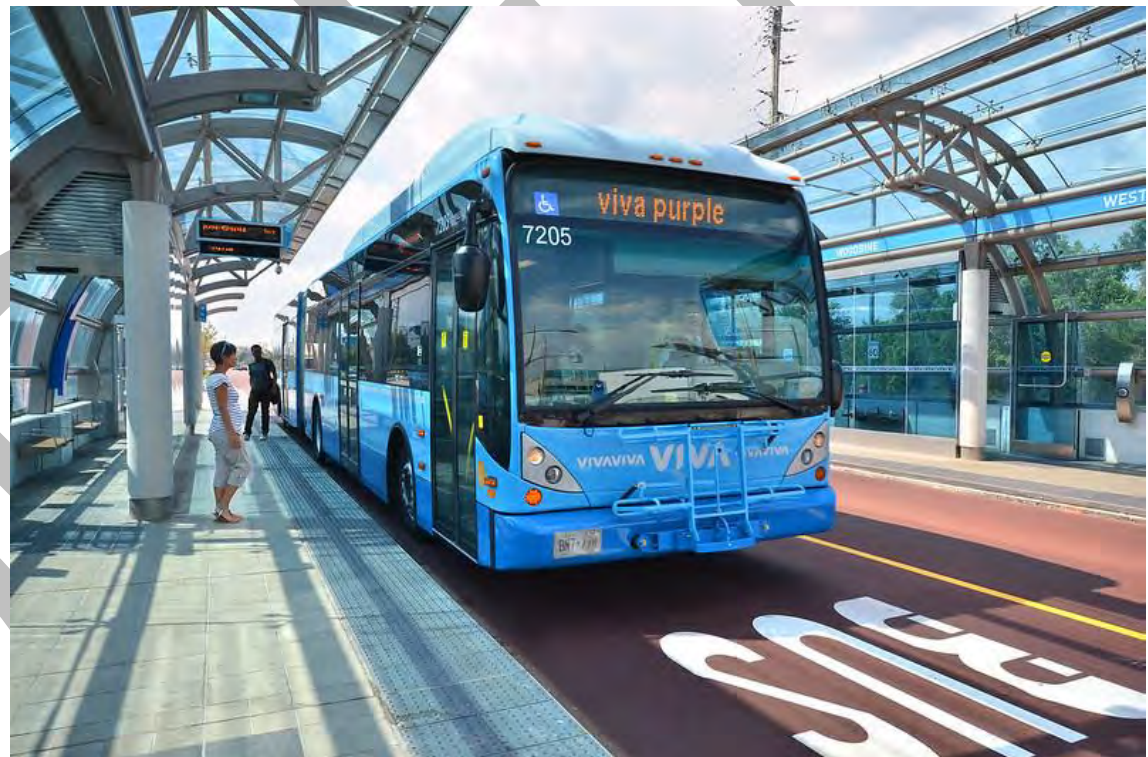
Figure 15 – Example of a BRT station Example of a Bus Rapid Transit (BRT) station - Ontario Growth Secretariat, Ministry of Municipal Affairs (2014)
