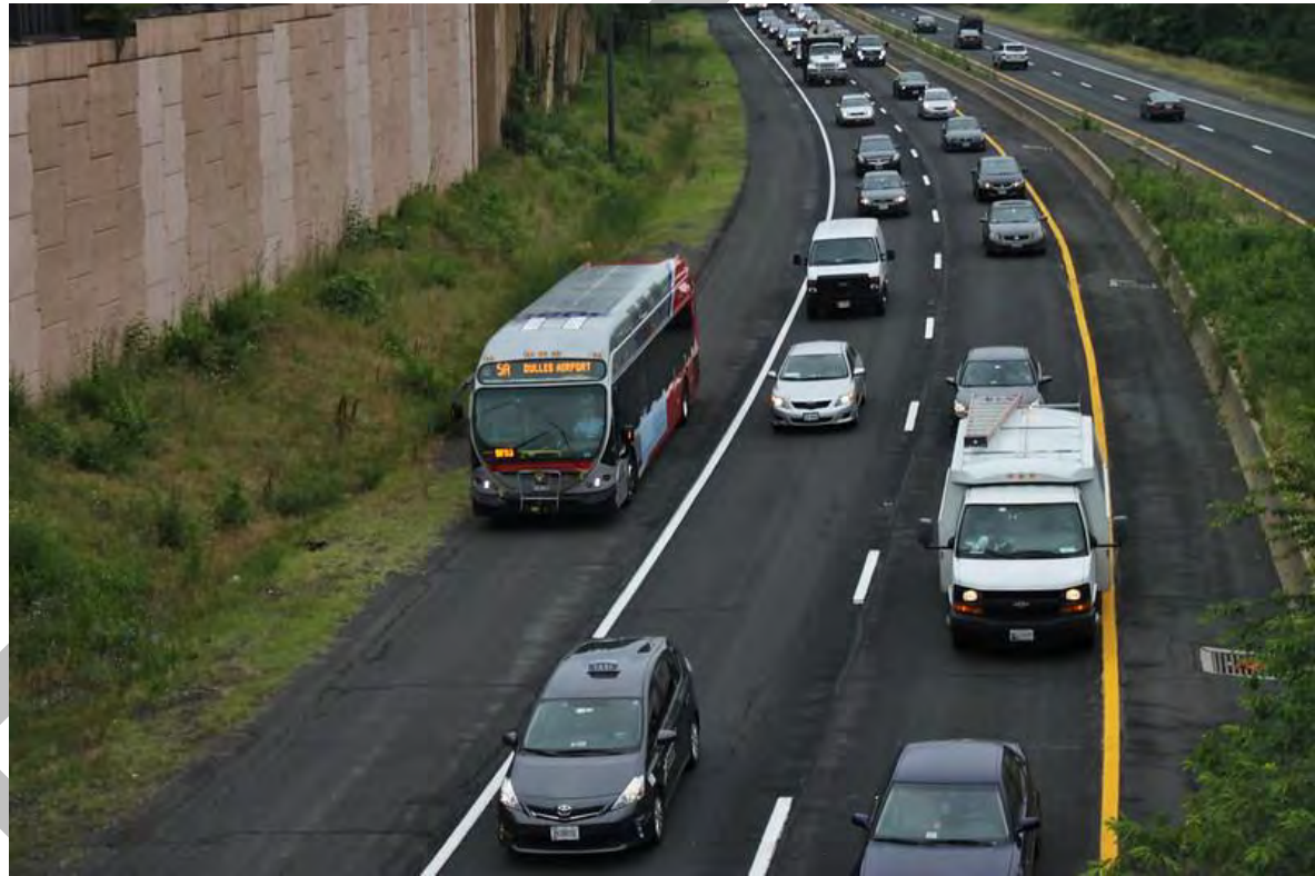
Figure 19 Example of transit bus using a highway shoulder lane “Metrobus shoulder bypass in Arlington, VA” by SounderBruce is licensed under CC BY-SA 2.0
